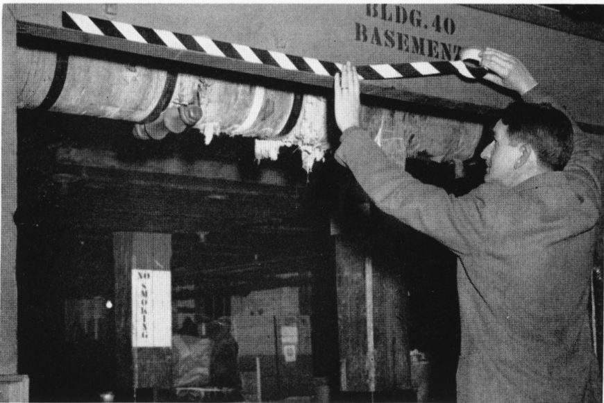
Bob Dobrick, Safety Dept. applies the latest in safety tapes to a low clearance doorway. Waterproof and acid resistant, this tape comes in various widths and can be easily applied to any clean surface to mark a hazard spot. The tape, when needed, may be obtained through the Safety Dept.
